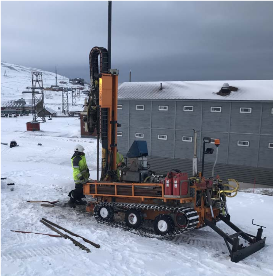
Figure 4 Drilling with Geotech 504.
