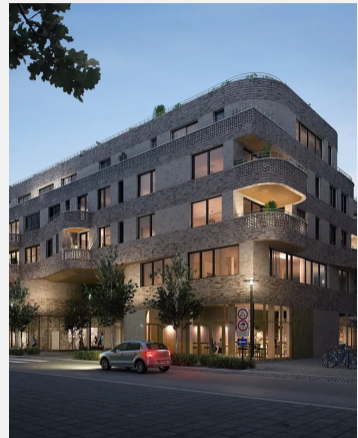
Residential/commercial building complex in Asker, Norway wesselkvartalet.no
