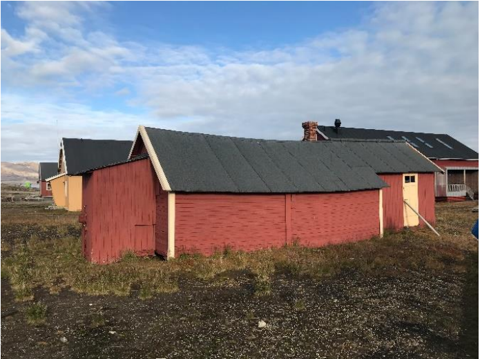
The Green Harbour house
