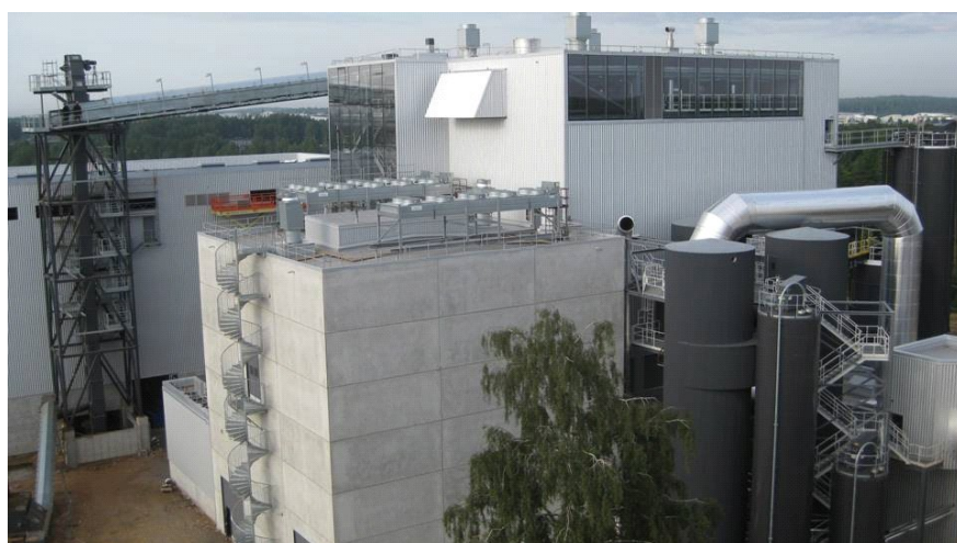
Figure 29: The Jordbro power plant (photo: Vattenfall)
