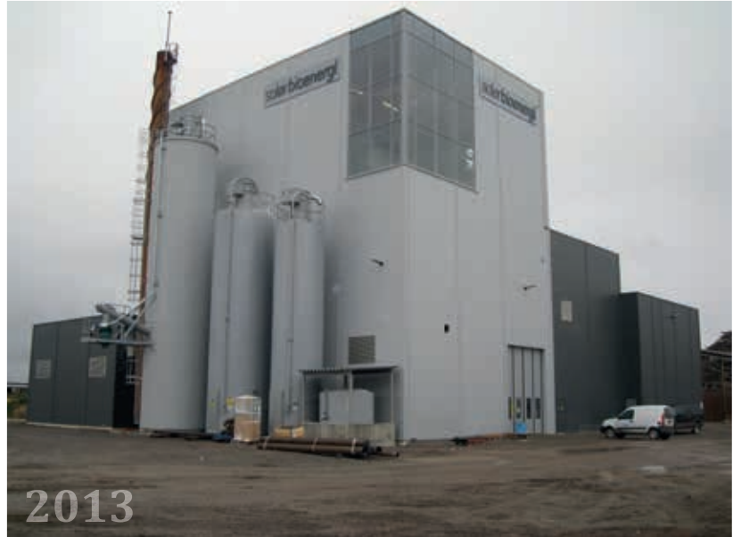
The Solør Bioenergi CHP plant. This plant processes impregnated wood waste to produce electricity, process steam and district heat. Photo: SINTEF.
