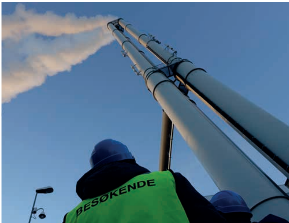
Chimneys of the Statkraft Varme Waste-to-Energy plant in Heimdal.
