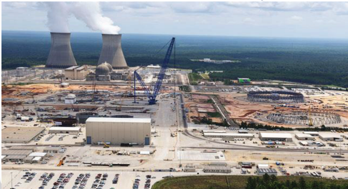
Plant Vogtle 3 and 4 construction site with Vogtle 1 and 2 in the background
