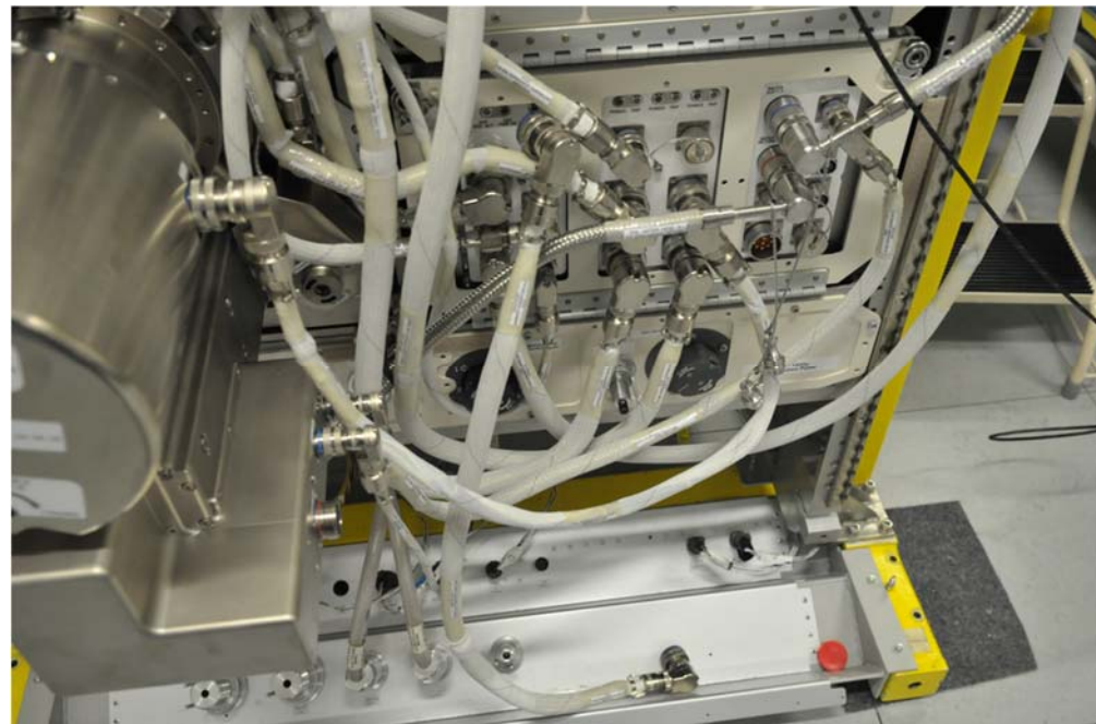
H/W installation check using a training model
