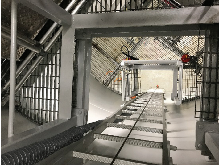
Figure 11: Working inside the tower
