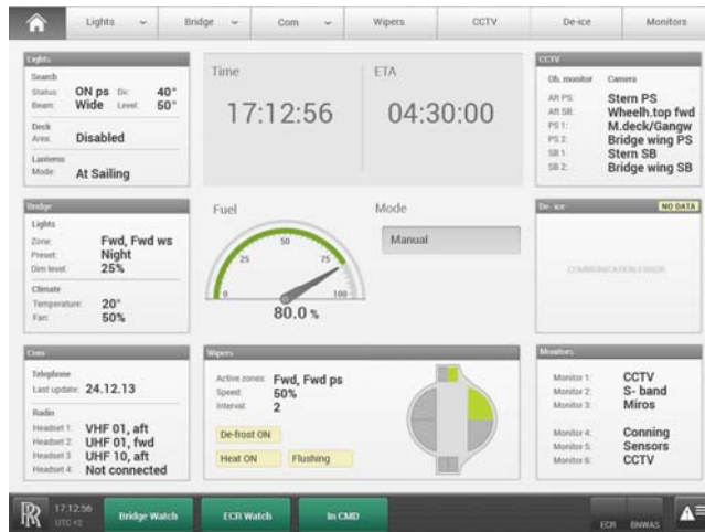
Auxiliary system running on 10" screen
