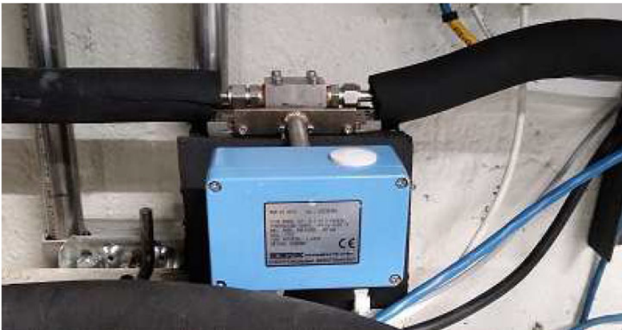
Fig 12 CO 2 cycle mass flow meter.
