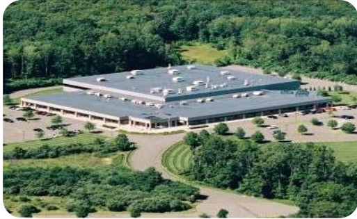
PEM electrolyzers Wallingford, CT, USA
