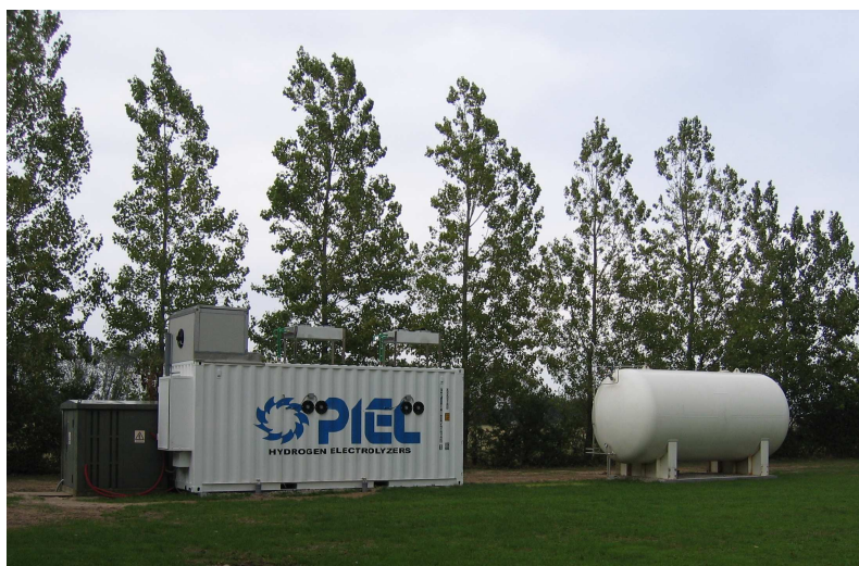
Fig. 4 Picture and key-numbers of the alkaline electrolyser installed in Vestenskov (project phase 2).
