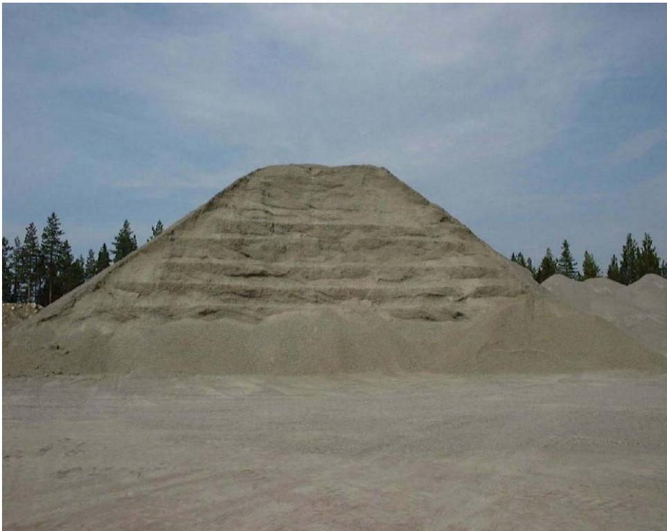
Figure 17: Aggregate stockpile made layer by layer.
