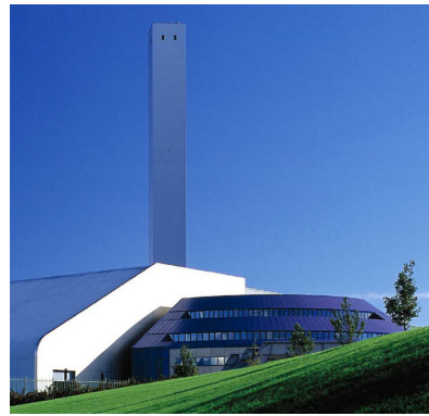
Brescia WTE plant
