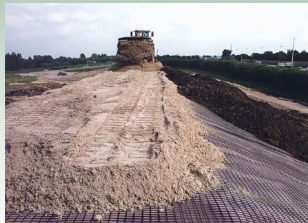
Utilization of MSWI bottom ashes as a road embankment material
