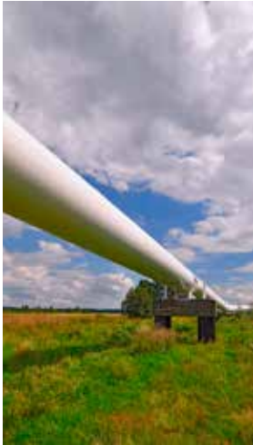
Natural Gas Pipeline Photo: Shutterstock
