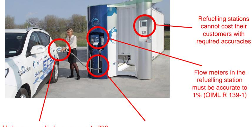
Hydrogen supplied can vary up to 700 bar in pressure and between -40 to 85°C during refuelling
