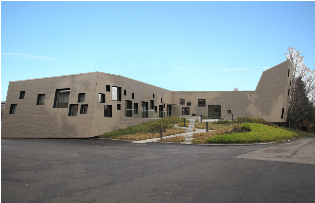
Tallhall – Norwegian Meteorological Institute in Oslo – Norway's first office building made of low-carbon concrete, opened June 2011. Architects: Pir II. Photo: SINTEF Building and Infrastructure
