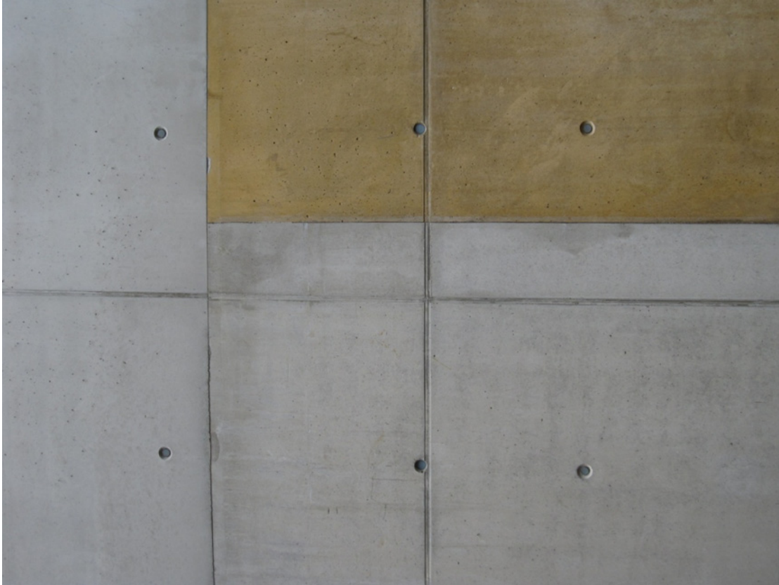
A smooth formed concrete surface ready to be classified.
