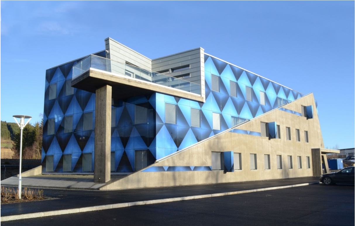
Veidekke's new regional headquarters in Rudshøgda, Hamar. Veidekke received the company's Concrete Prize 2012 for this building. Photo: Veidekke
