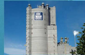
Yara Porsgrunn Ammonia production
