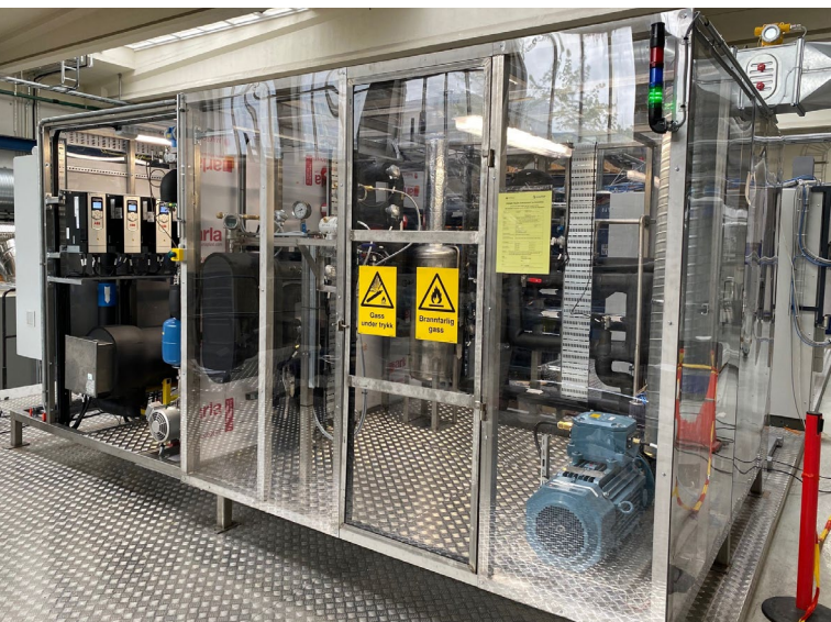
Heat exchanger test rig – HighEFFLab.
