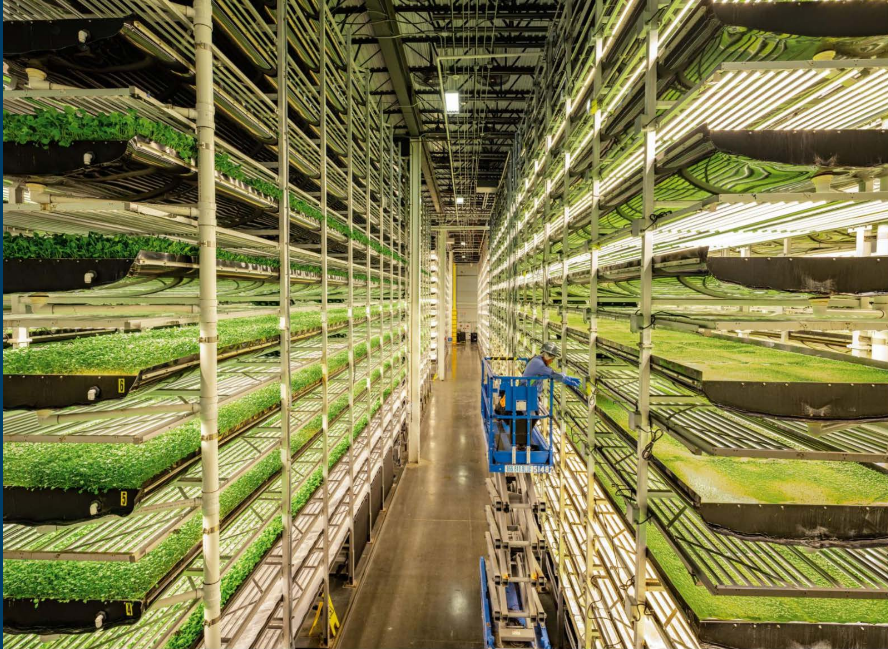
The world's largest indoor vertical farm, operated by AeroFarms at its headquarters in Newark, New Jersey, aims to raise vegetables sustainably year-round in the heart of cities. Baby leafy greens are grown on a reusable substrate made from recycled plastic bottles. Water is misted on the roots from below, saving 95 percent of what would be needed outdoors. No pesticides are used. Nutrients and fertilizers are applied only as needed. And the lighting provides the specific wavelength that the vegetables require. The company says its yields are 390 times as high as farming in fields.
