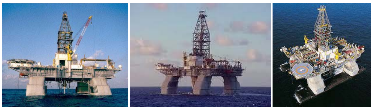
Figur 2.1 Boreinnretningen Deepwater Horizon (Foto: Transocean / Rigzone).
